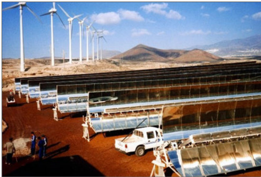
Figure 5: Parabolic troughs, like those used in this Euclides-Thermie installation in Spain, concentrate sunlight onto a strip of high-efficiency solar cells positioned above the troughs.
