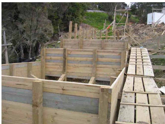
Figure 8: Cascading runoff treatment structure (under construction) at Verbena Road
