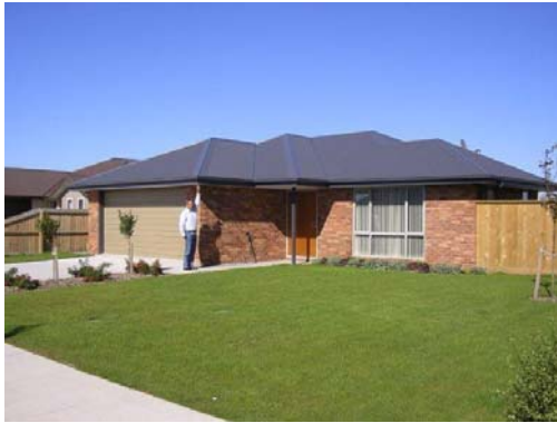
Figure 2: EnerG Wall home
