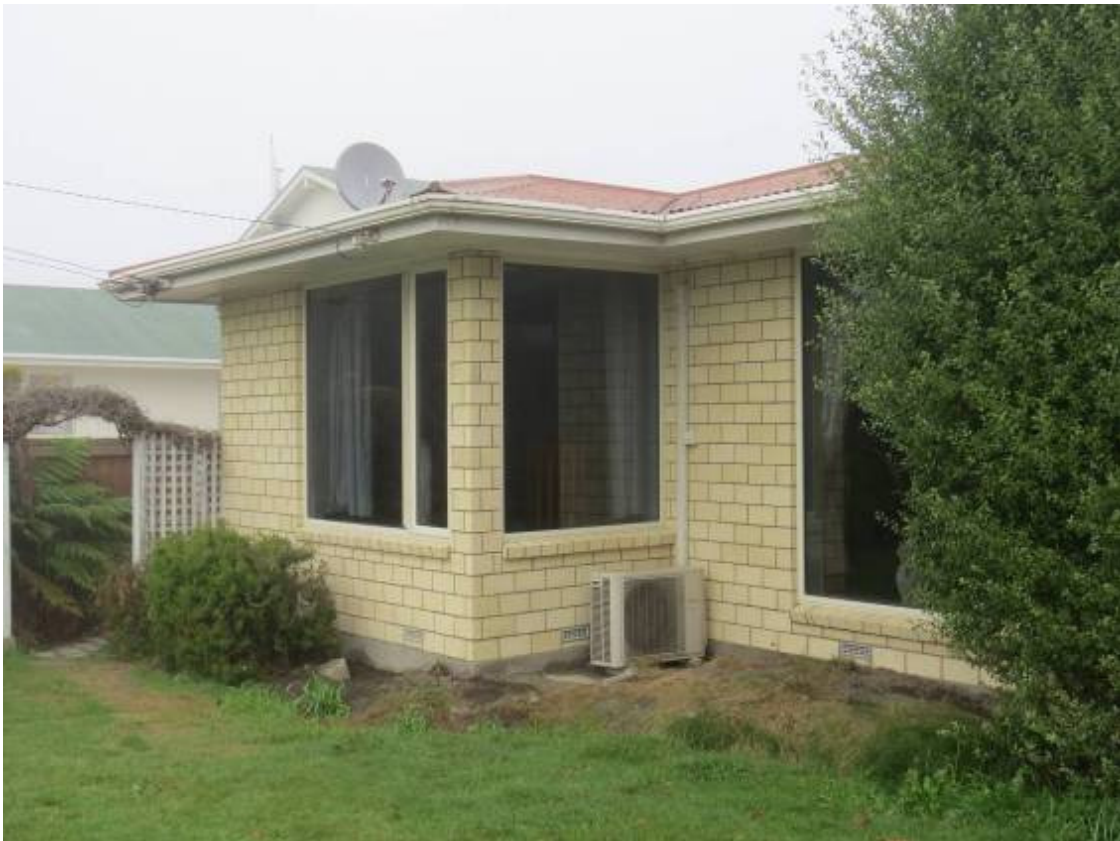
Figure 10: Completed brick veneer replacement and new double glazed windows installed at homeowner's cost.
