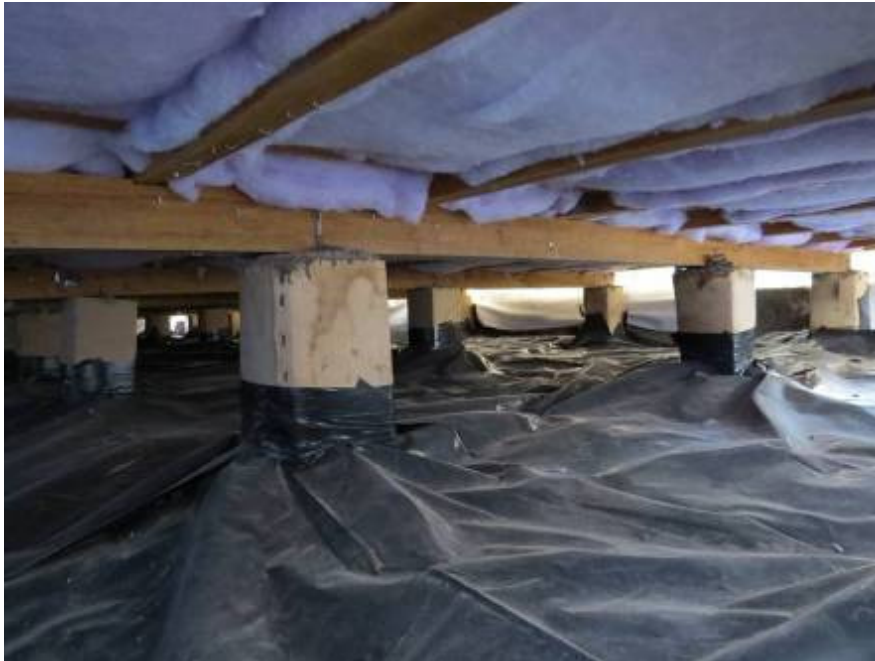
Figure 8: Ground vapour barrier and underfloor insulation While the liquefaction was removed from under the house, substantial dampness remains. The ground vapour barrier is a critical intervention to prevent the return of mould and excessive moisture into this house.
