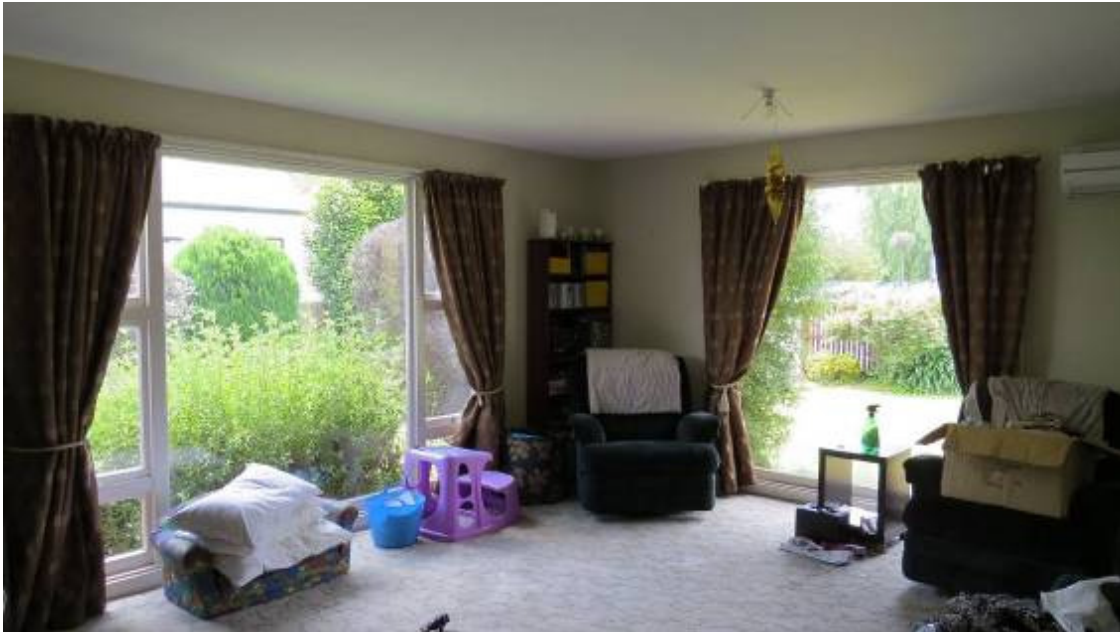
Figure 4: Large draughty windows facing north and west causing overheating in Halswell 1
