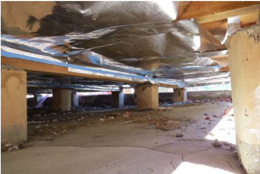
Figure 3: Contaminated liquefaction under Halswell 1
