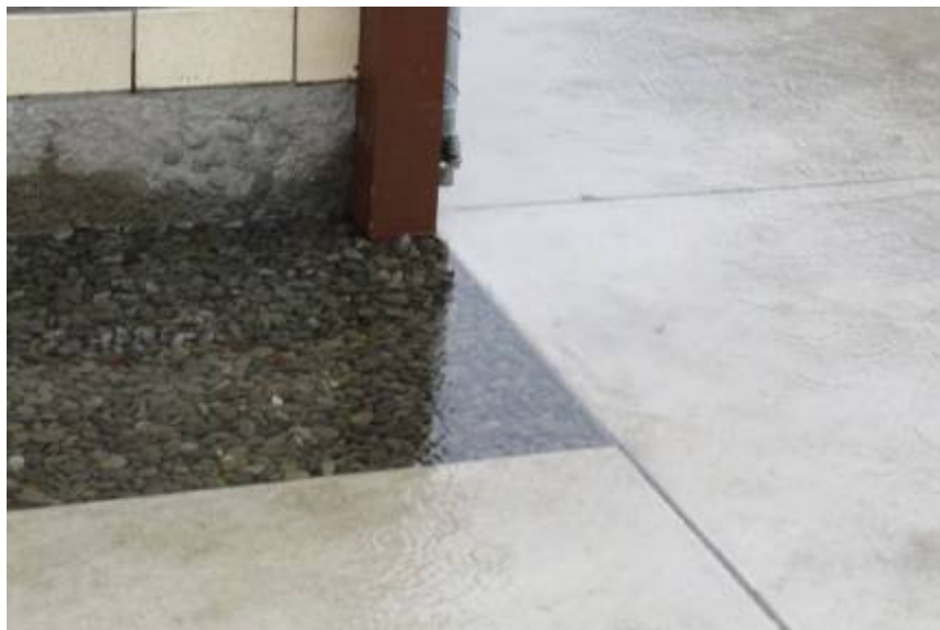
Figure 7: Post completion flooding on the driveway during June 2013 floods The combination of too much paving, absence of drainage systems and ground subsidence means this home will always have issues with stormwater during heavy rain events.
