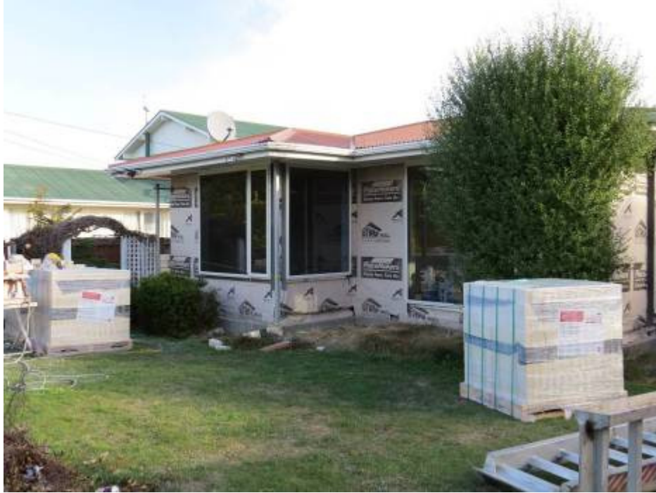
Figure 6: New windows installed while cladding was removed – a classic Build Back Smarter opportunity
