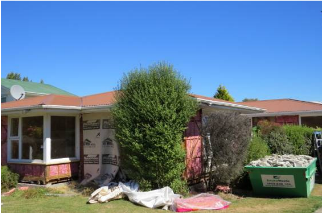
Figure 5: Mid-repair – Wall insulation being installed from the outside prior to building wrap and recladding
