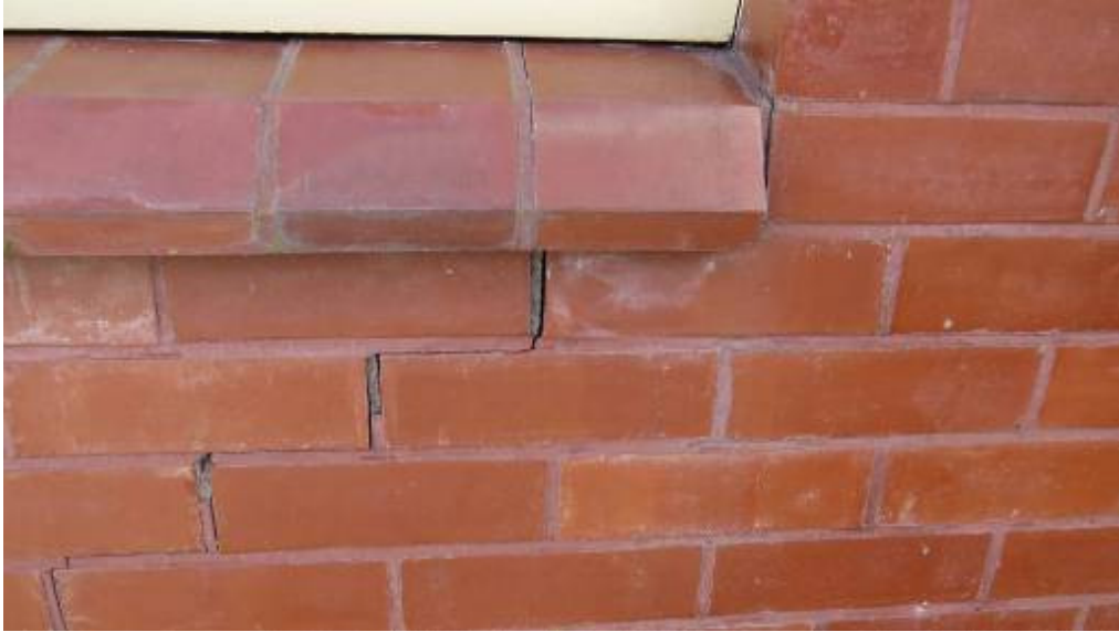
Figure 2: Earthquake damage to Halswell 1 exterior cladding
