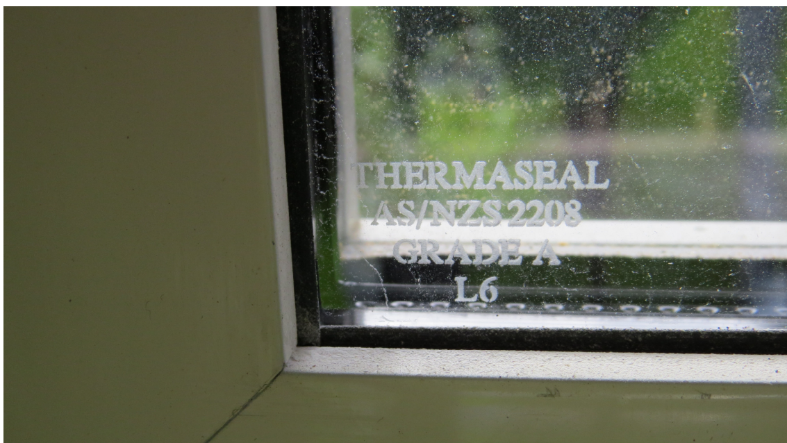
Figure 9: Double glazing with thermally broken aluminium frames, low emissivity and argon filled glass with a glare tint in living areas
