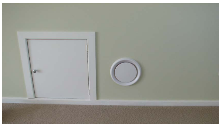
Figure 12: An access hatch to install ceiling insulation, and heat transfer kit to the master bedroom were installed as part of the upgrade.
