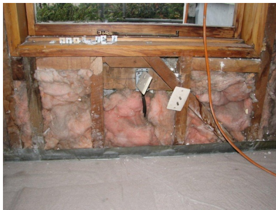
Figure 6: Old insulation in the living room walls (this wasn't expected but was replaced as part of the Build Back Smarter work)
