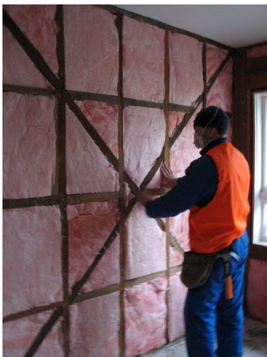
Figure 7: Wall insulation being installed prior to relining
