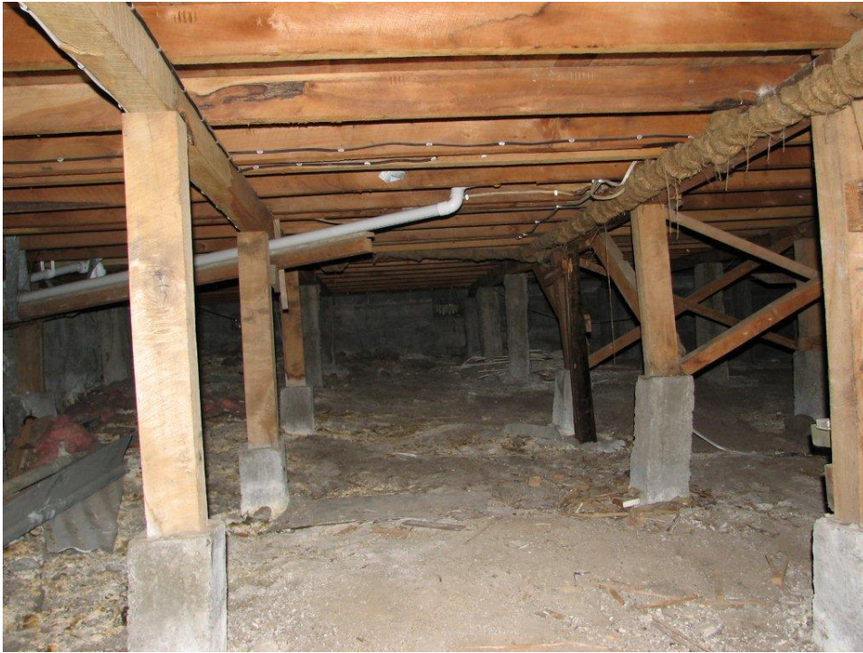
Figure 3: Uninsulated suspended timber floor in Huntsbury 2
