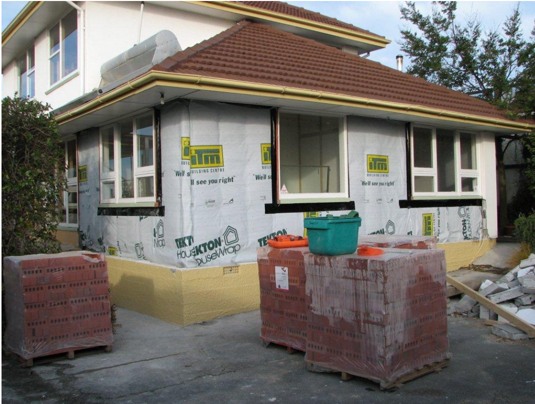
Figure 4: Huntsbury 2 mid repair – Exterior cladding being replaced
