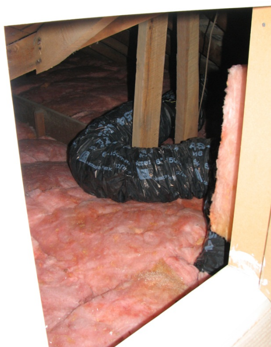
Figure 8: Ceiling insulation topped up with heat transfer system also installed
