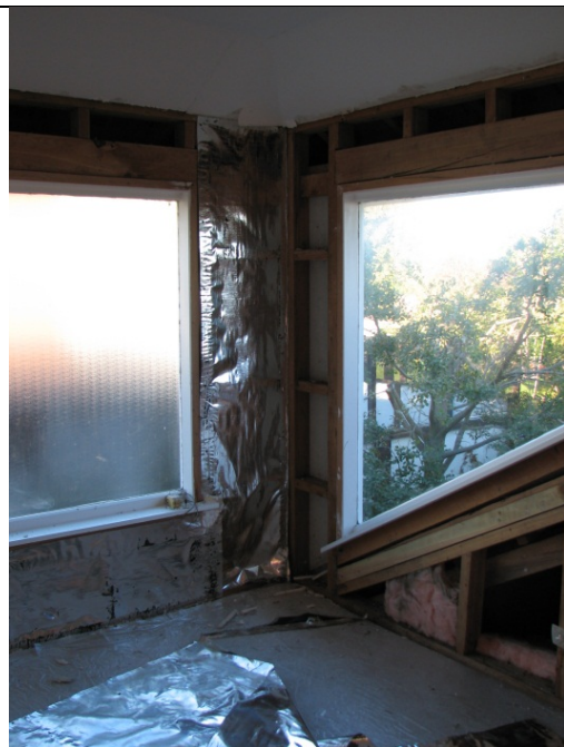
Figure 9: Foil sheet behind plasterboard was found in the upper storey when the linings were removed.
