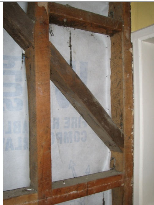
Figure 10: Inserts of building paper were stapled into the cavities prior to insulation installation where wall linings, but not cladding, were replaced
