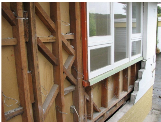
Figure 5: Uninsulated wall with cladding removed – a classic Build Back Smarter opportunity
