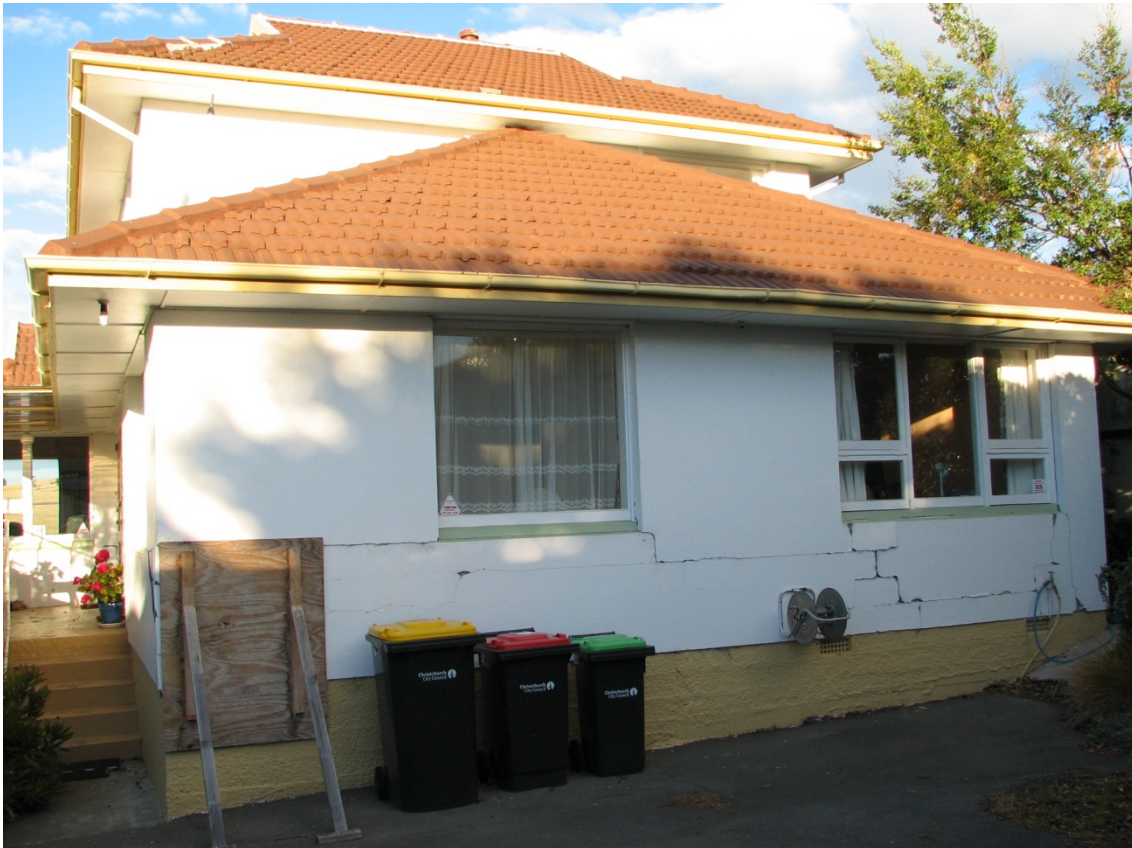
Figure 2: Earthquake damage to Huntsbury 2 exterior cladding
