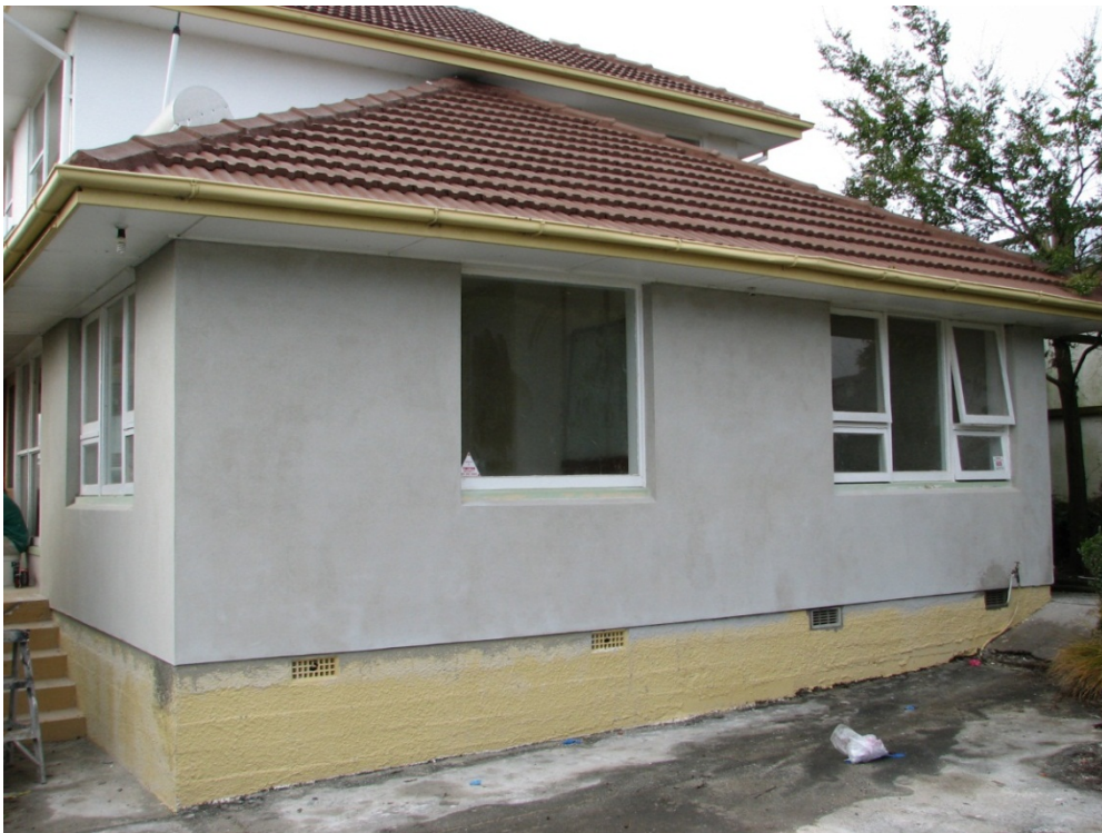
Figure 11: Completed stucco block veneer replacement – additional fibreglass reinforcing was included at the homeowner’s cost
