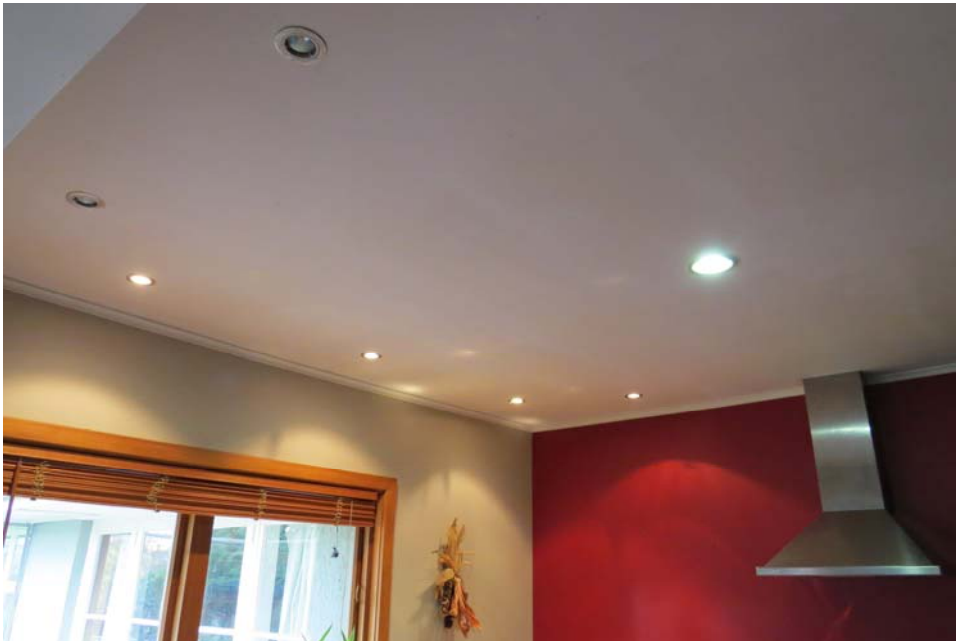
Figure 3: Extensive downlights were replaced with LED/IC-F rated downlights
