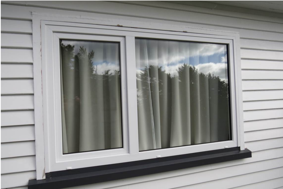
Figure 7: Windows were replaced with double glazed uPVC windows at the homeowner's cost.
