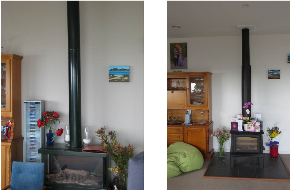
Figure 3: A gas effect fire (left) replaced by woodburner (right)
