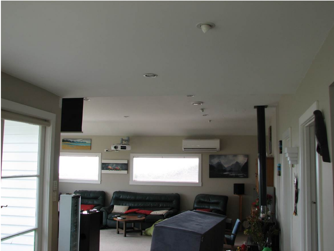
Figure 5: Downlights were widespread in the house with halogen and incandescent bulbs.
