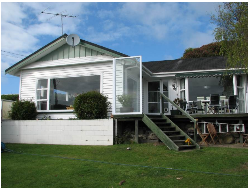
Figure 4: Extensive north-facing glazing to take advantage of the views has led to overheating – some awnings already installed
