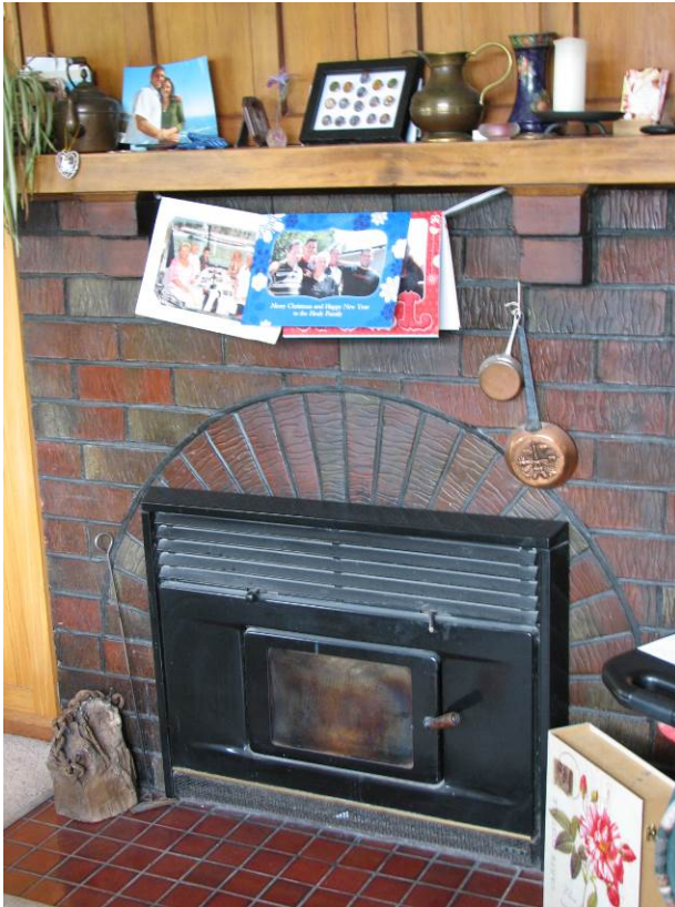
Figure 5: An old inset wood burner with a wetback was replaced with a modern freestanding woodburner, wetback and new hot water cylinder.
