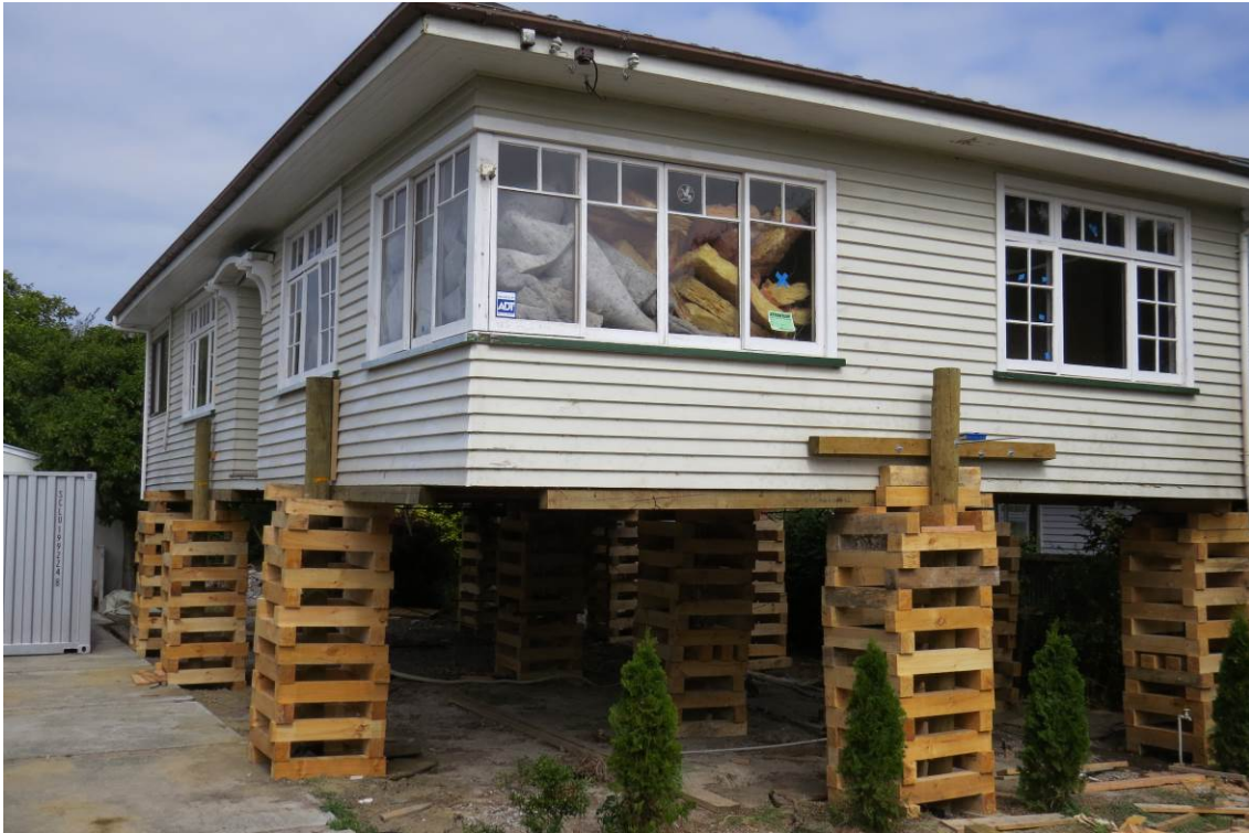
Figure 3: The house was lifted up for foundation repair – enabling access to install underfloor insulation and a ground vapour barrier in Spreydon 1
