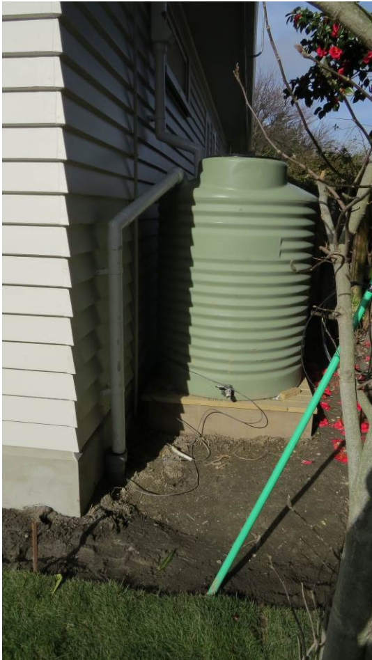
Figure 11: A 1000 litre rainwater tank was installed as part of the water retrofit measures
