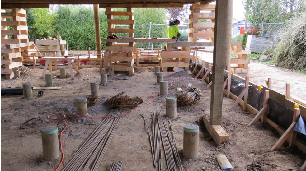
Figure 6: A new system of installing pile foundations was trialled by the repairer of Spreydon 1.
