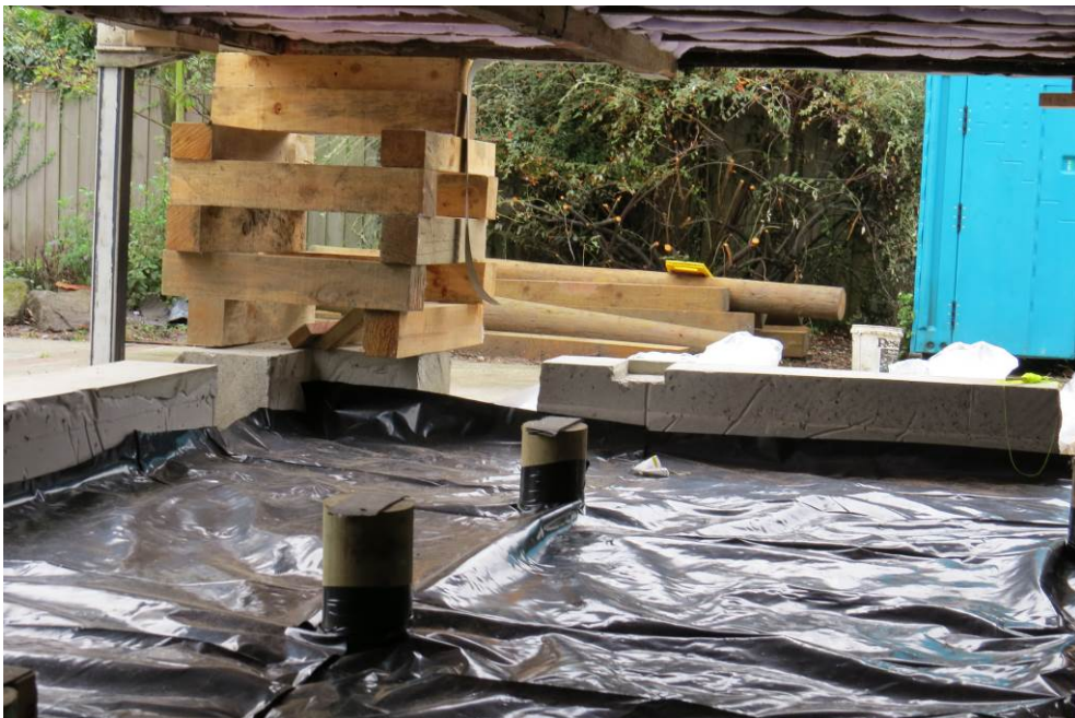
Figure 7: Lifting the house up to replace the foundations enabled easy access for both underfloor insulation and ground vapour barrier installation for this previously cold and damp house underfloor
