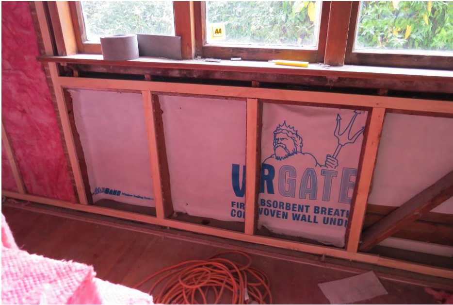
Figure 8: Building wrap inserts were stapled into the framing as part of the wall insulation installation process
