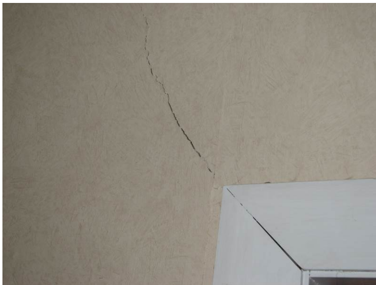
Figure 2: Earthquake damage to Spreydon 1 wall linings
