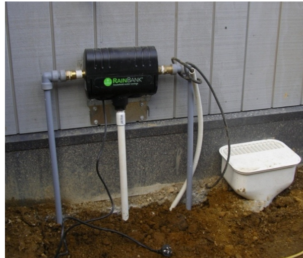
Figure 12: The Rainbank rainwater tank controller during construction
