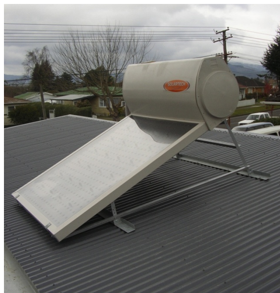
Figure 3: The flat plate thermosiphon SWH system in the Rotorua NOW Home®
