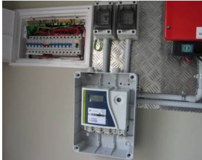
Figure 8: Installation of the Energy Intellect™ meter
