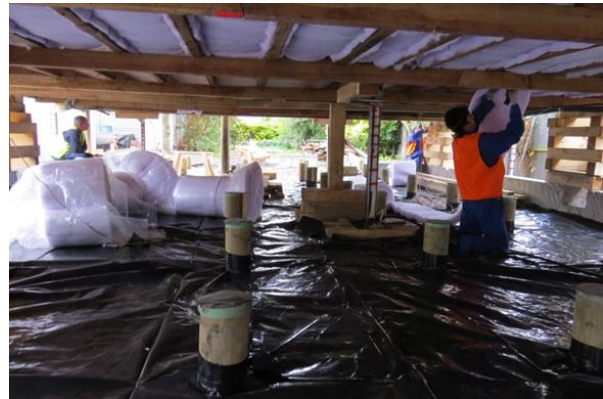
While lifted, both underfloor insulation and a moisture barrier were installed.
