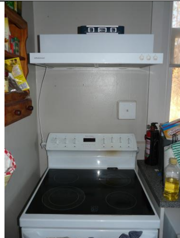
A range hood which covers the stove area is much more effective
