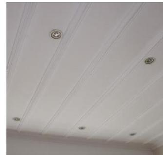
Additionally, downlights in wet areas, like bathrooms and kitchens, can allow moist air into roof spaces and around concealed framing, resulting in condensation and possible moisture damage.
