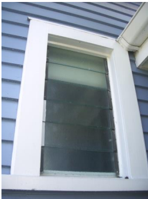
A draughty louvre window is replaced by secondary glazing – aluminium inserts placed into the wooden frames
