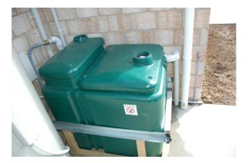
when they left the house for several days. On average, the system saved 23 litres of water per person per day, reducing household use of reticulated water by 20%. It also removed 115 litres of wastewater per day from the waste stream and used 68 kW of electricity over a one year period.
