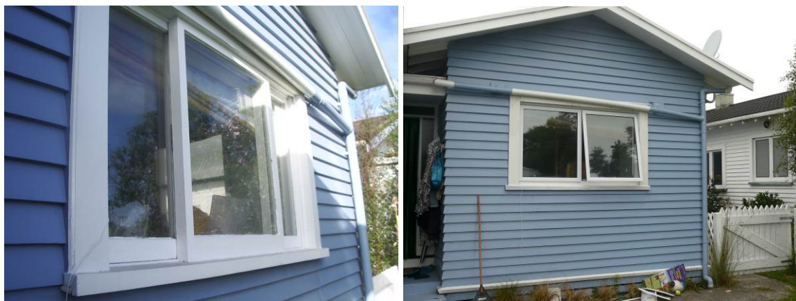
Before and after double glazing the bedroom window
