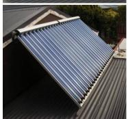
The Papakowhai panels sat at 41° to match the latitude of the site. With large collectors and cylinders, these systems provided 75% of hot water.
