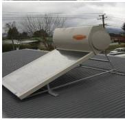
The Rotorua NOW Home panel was limited to 30° by the framing that it came with. It should have been at 38°. This system provided only 36% of water heating. The outdoor cylinder also had the most heat loss.
