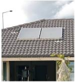
The Waitakere NOW Home panels were only installed at 20° in line with the roof. It should have sat at 37°. This system provided only 45% of water heating.
