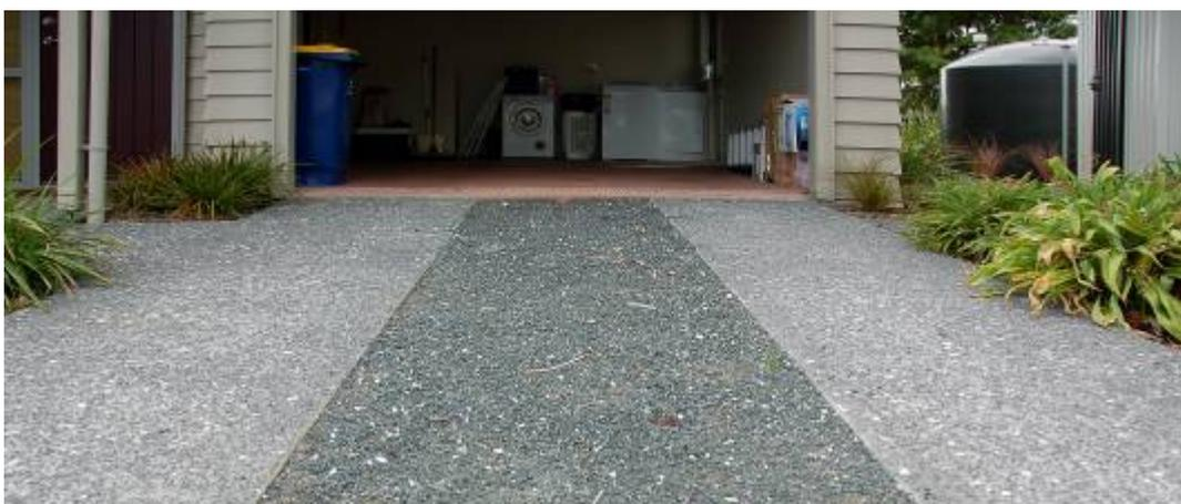
Concrete strips with gravel allow more stormwater to soak into the ground during rain
