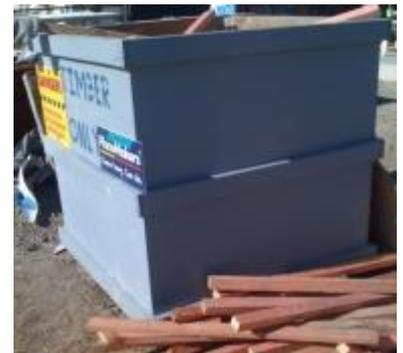
Off-cuts and other construction waste were sorted and weighed on site. Where possible, materials were re-used or recycled, and only the remaining materials were sent to the landfill.
