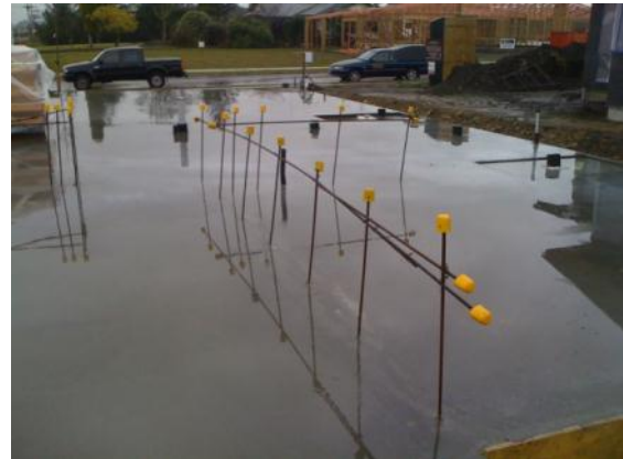
Concrete slab with reinforcing for thermal wall
