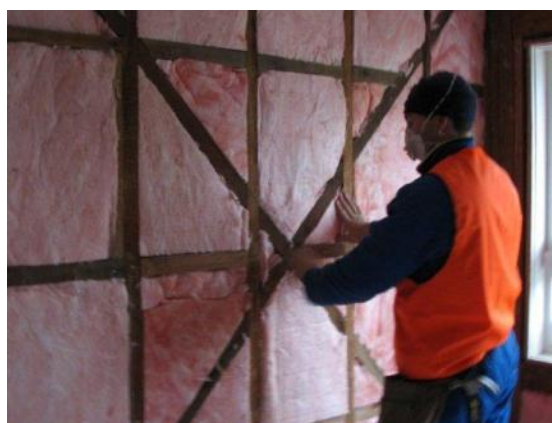
CEA worker installs new insulation
