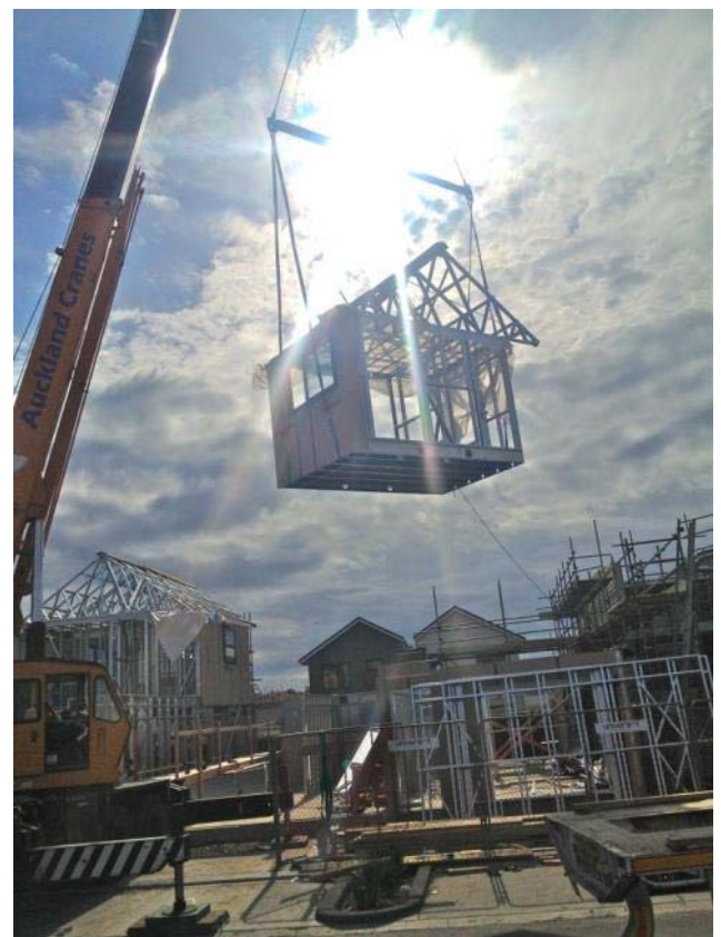
An upstairs module gets craned into place.
