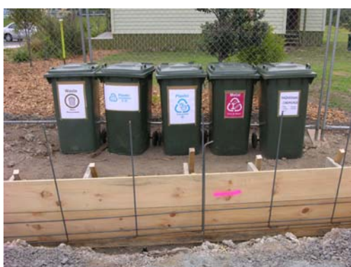
Sorting construction waste during the construction of the Waitakere NOW Home®
