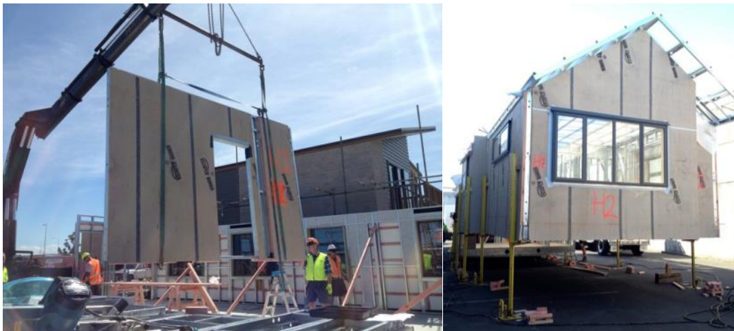
2D walls (left) vs 3D modules (right)
